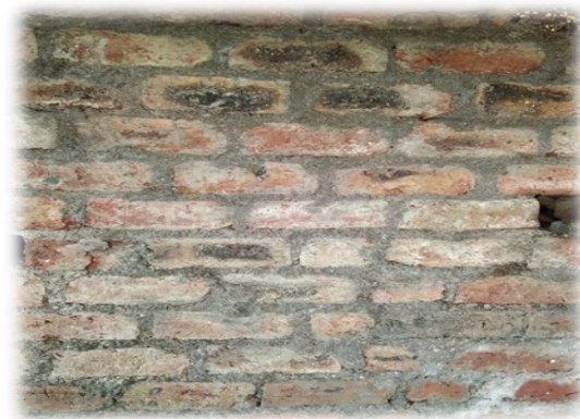
Brickwork on site in Stretcher Bond
